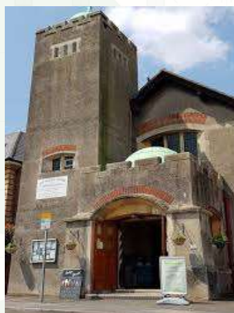
The Village Centre (1902) – Grade II
