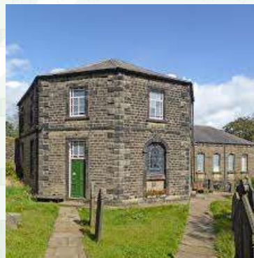
Cautley, Sedbergh (1845) - Grade II
