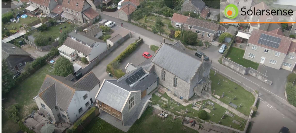
Pilton Methodist Church – Grade II Solar slates & solar array on new extension
