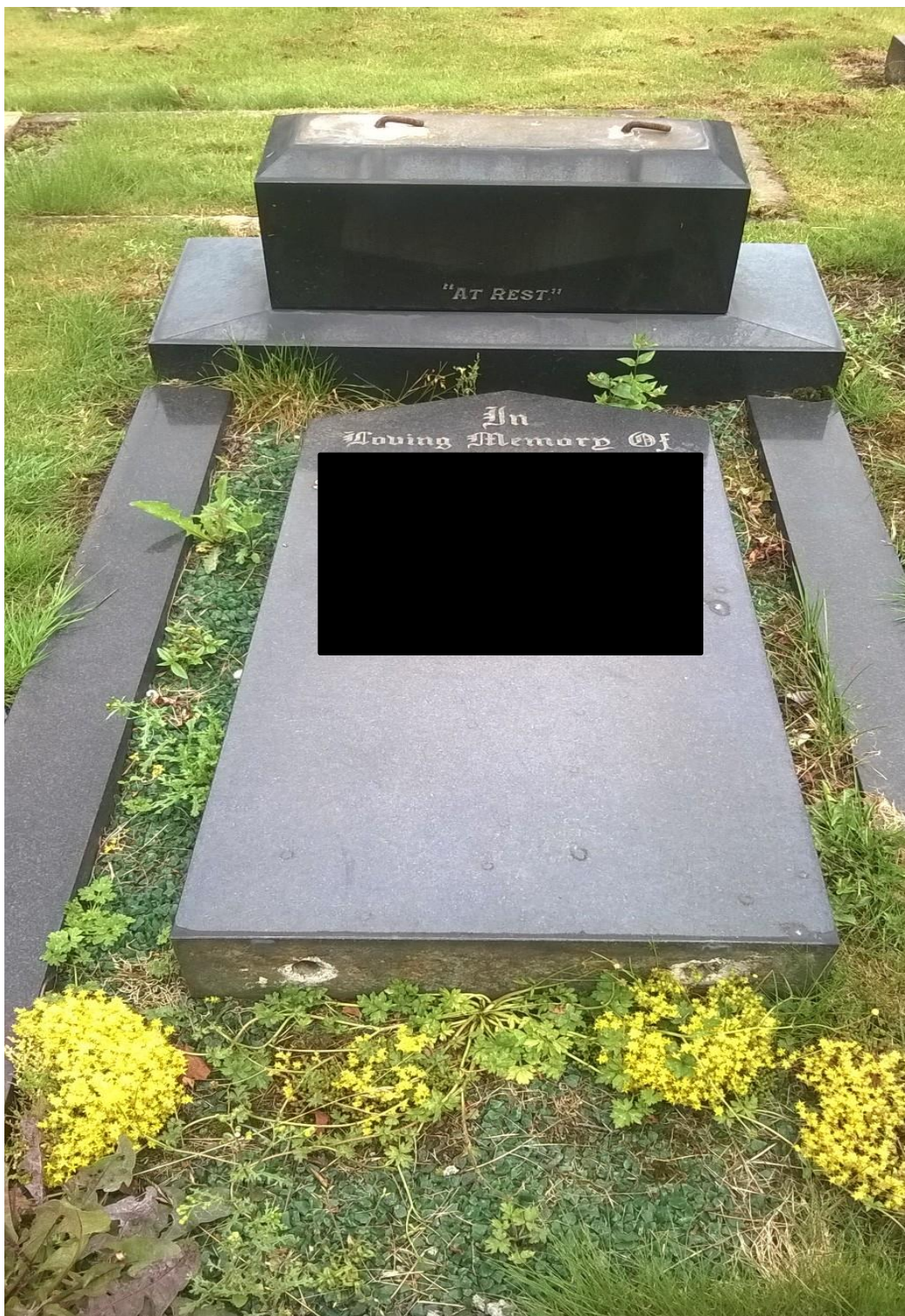
Example of an unsafe memorial laid flat in between existing kerb sets.
