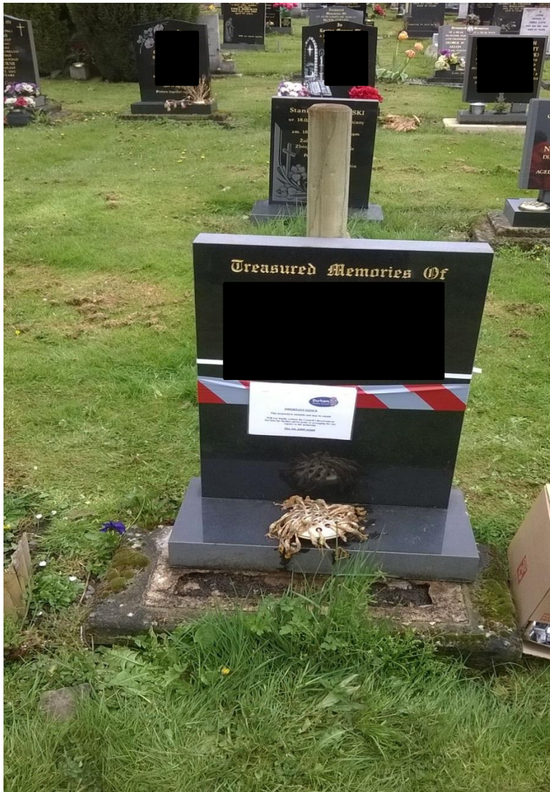
Example of a warning tape notice and banding attached to an unsafe memorial.
