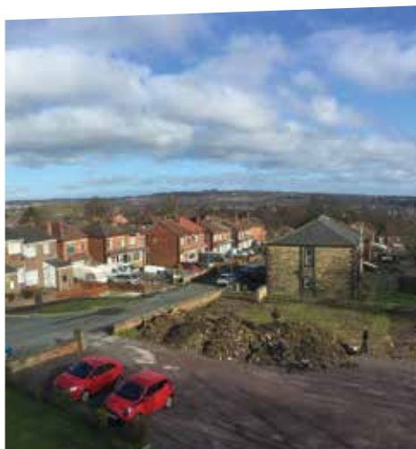
The site in the early stages of clearance
