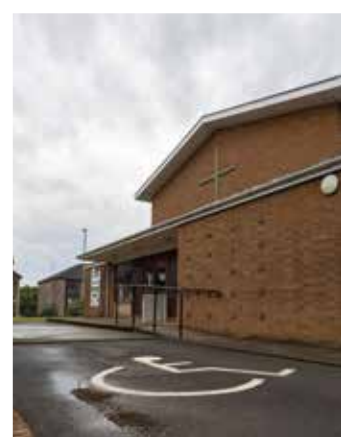
Improved access into the church
