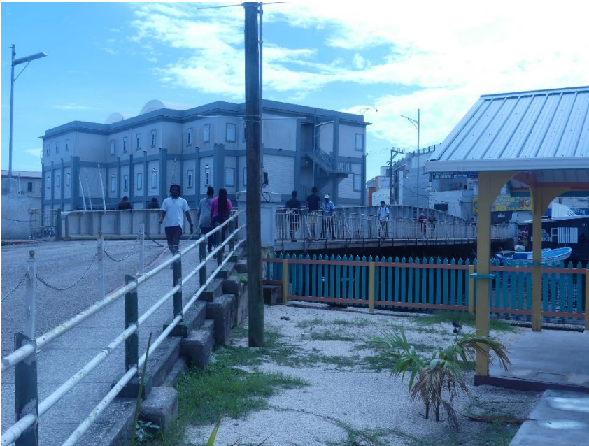
Swing bridge, Belize City
